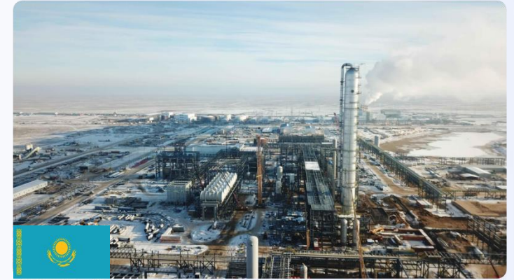
Kazakhstan Petrochemical Integrated Plant
