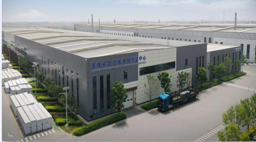
Prefabricated Truss Deck Manufacturing Center
