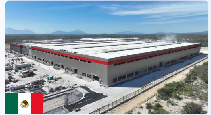
Mexico LGMG industrial park
