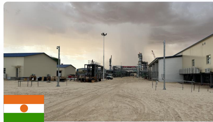
Niger oil field construction project
